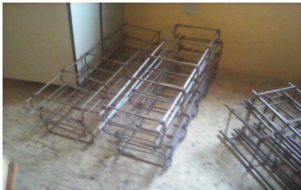
Plate 3.3: Beam reinforcement cage with shear
