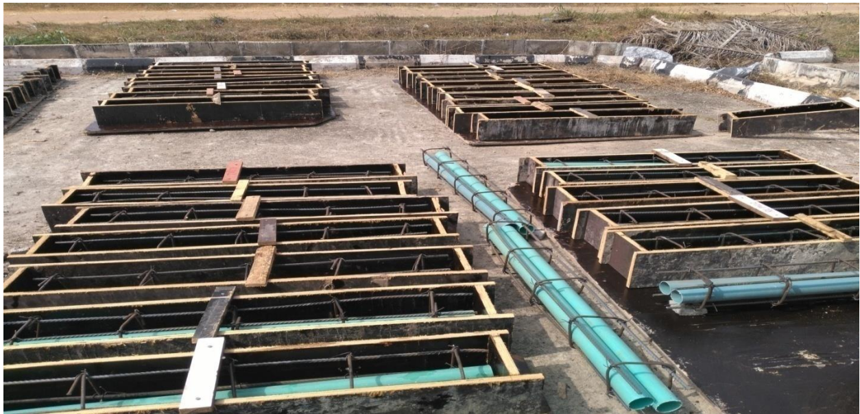
Plate 3.15: Formwork preparation for normal concrete and concrete with embedded PVC
