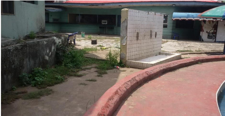
Plate I: State of Facilities at Water Park in Allen Avenue, Ikeja Source: Field Survey, 2016
