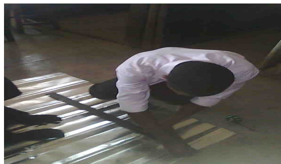
Figure 4 Marking out the roofing sheet
