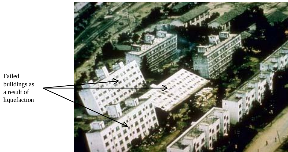
Figure 2.3: The Kwangishicho Apartments in Niigata Japan being tilted due to liquefaction Ammon 2005
