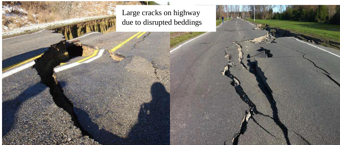
Figure 2.7: Disrupted bedding effect on highways Schierle 2003
