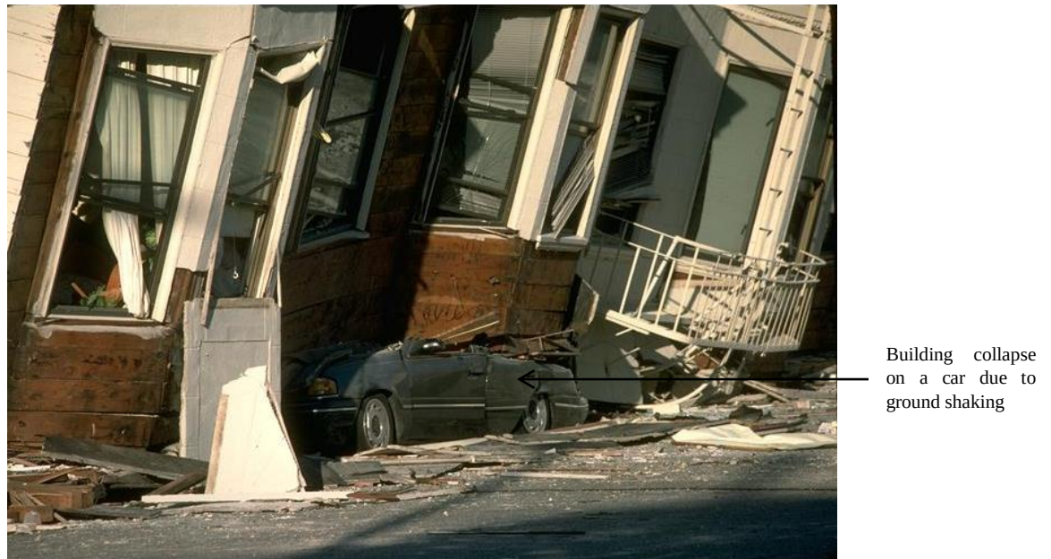
Figure 2.1: A damaged building from the Marina District in San Francisco after the Loma Prieta earthquake in 1989 Anderson 1997
