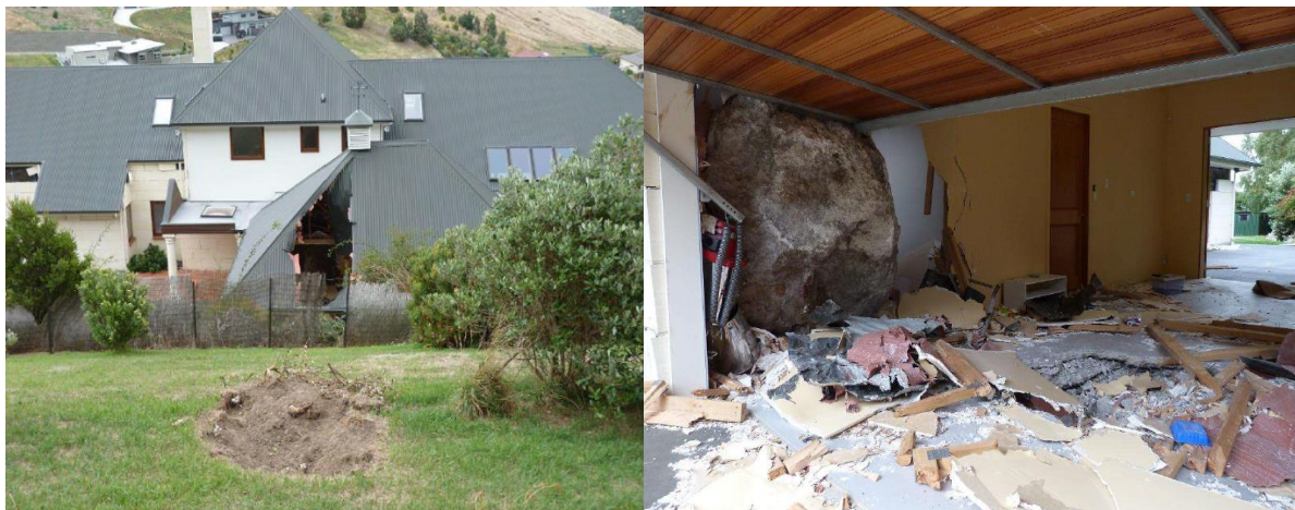
Figure 2.11: A fallen rock inside a building Ammon 2005
