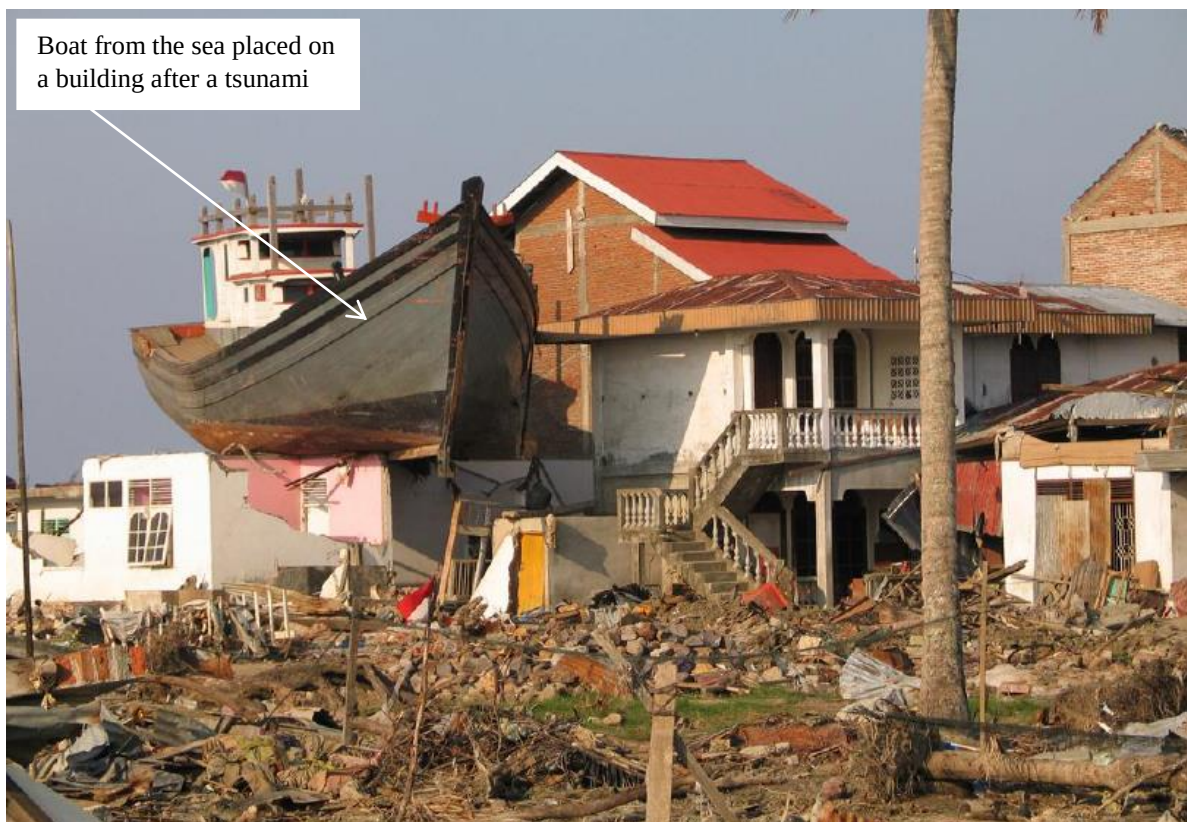
Figure 2.9: Damages after the Sumatra Tsunami Ammon 2005
