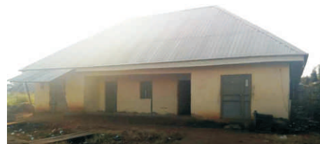
Plate 7: A compound of 14 single rooms. (Source: Authors Field Work)
