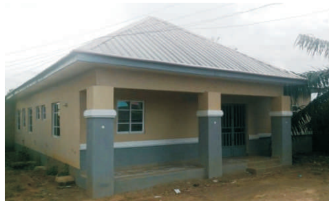
Plate 8: A compound of 8 single rooms, redevelopment, (Source: Authors Field Work)
