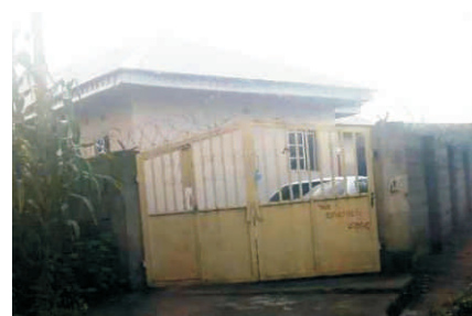
Plate 3: A new development of 6 fully en-suite apartments on a farmland. (Source: Authors Field Work)
