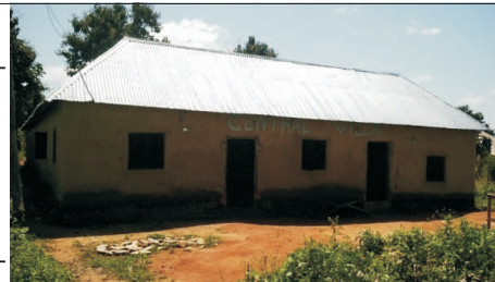
Plate 5: A compound of 16 single rooms (Source: Authors Field Work)
