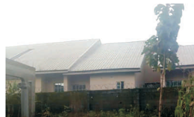
Plate 2: A new development of 8 fully en-suite apartments on a farmland. (Source: Authors Field Work)
