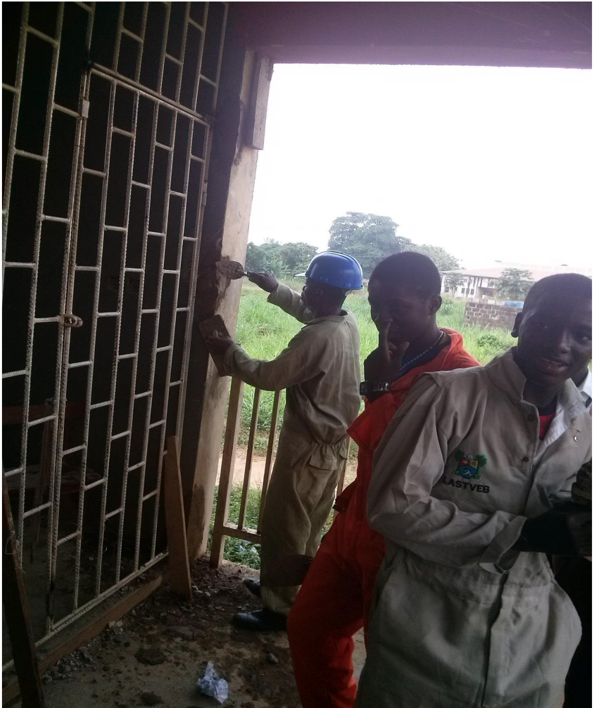
Students and their instructor in bricklaying and concrete skills session at GTC Ikotun
