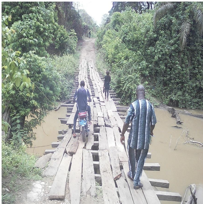
Figure 30: Another bridge linking Onyuwei to the major Otobi road (Researcher: 2017)
