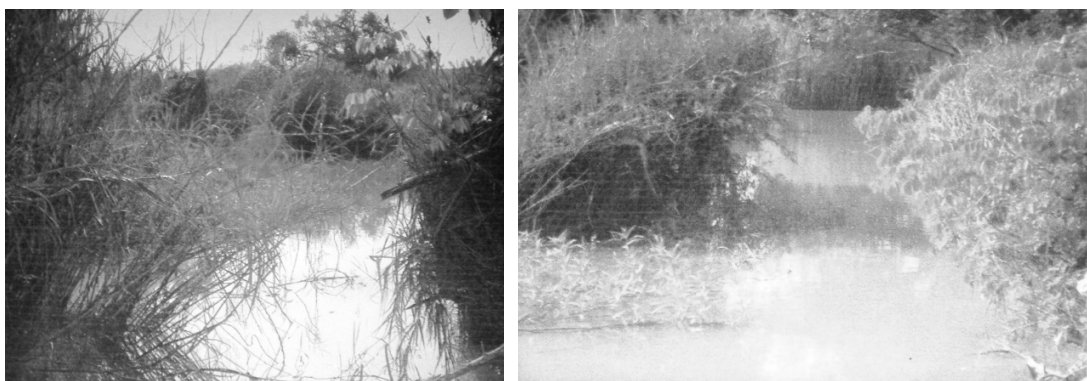
Figure 1 River channel overgrown with vegetation at Ch 3 + 300 and Ch 4 + 800
